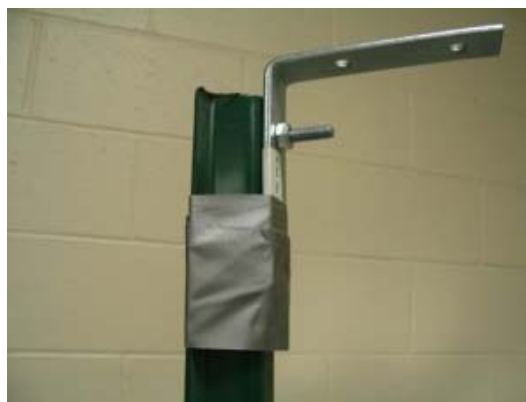
Figure 6 – L-bracket attached to fence post, with duct tape.
