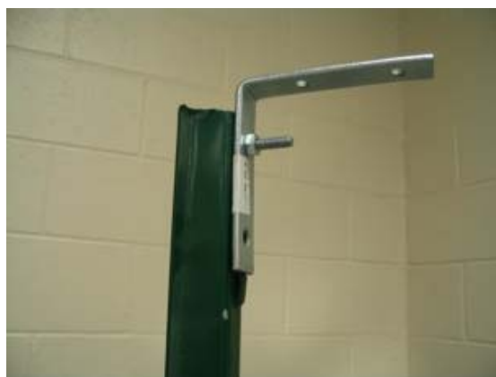
Figure 5 – L-bracket attached to fence post.
